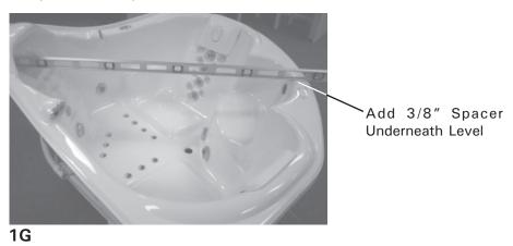
3. After leveling the front to back of the whirlpool, check the left to right level. If not level, re-adjust until level. Check again until left to right and front to back are both level.
